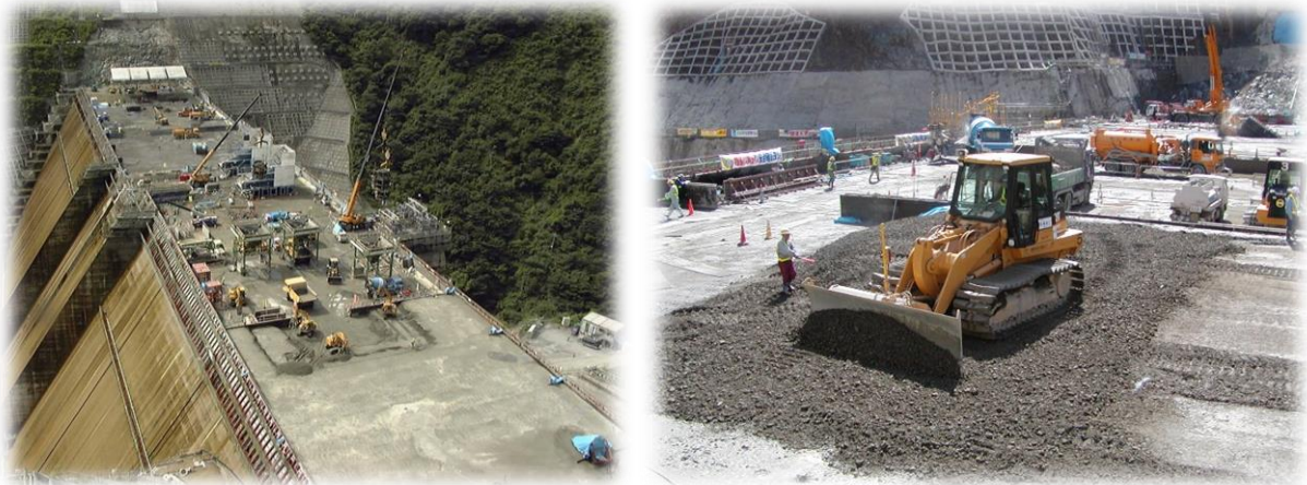
Photo 4 : Photo of the control stage of the Takizawa Dam
