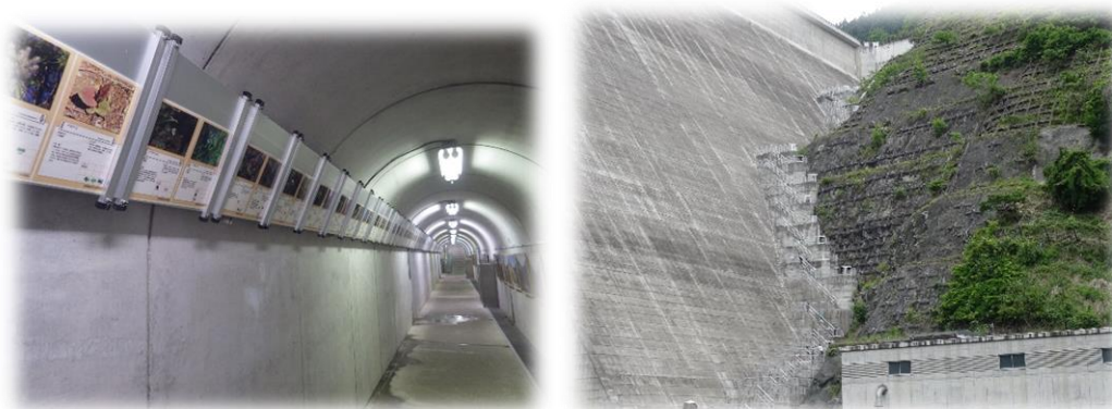
Photo 8 : Corridor of the inside of dam body and 435 steps on dam body
